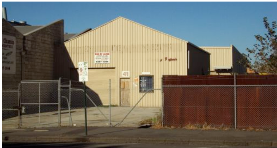
Figure 19 Vacant auto repair workshop at 41 Nelson Place (part of Lot 3).
