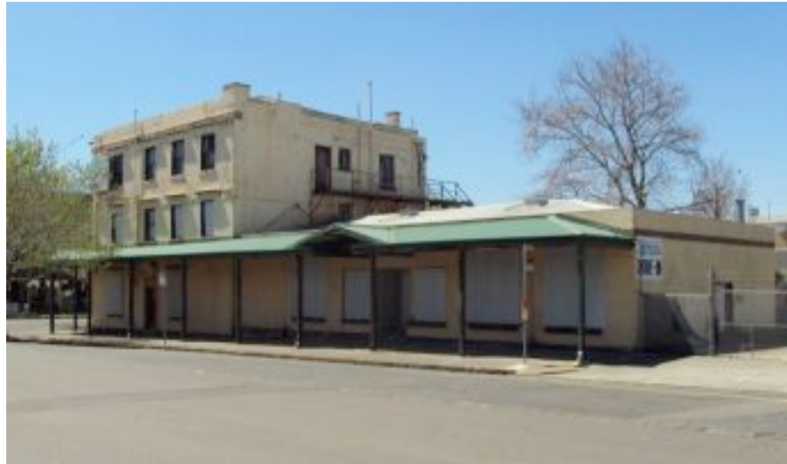
Figure 16 The Ann Street elevation showing modern single-storey wing and verandah to the south of the corner three storey building.
