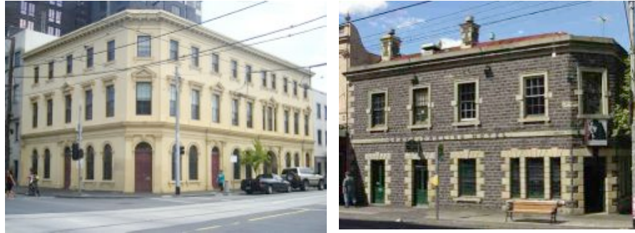
Figure 36 (left) Former Eastern Hill Hotel, Victoria Parade, Fitzroy. Built c1854-1856, this substantial three-storey hotel demonstrates the impact of the gold-rushes on Melbourne's development (VHR816).
