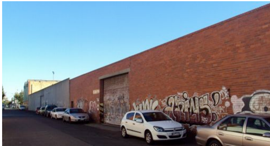
Figure 22 The Aitken Street frontage of the subject site looking west from Kanowna Street.
