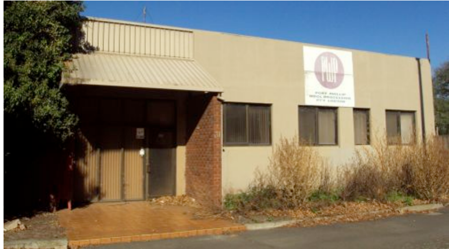
Figure 18 Former Port Phillip Woollen Mills office building on Nelson Place (part of Lot 3).
