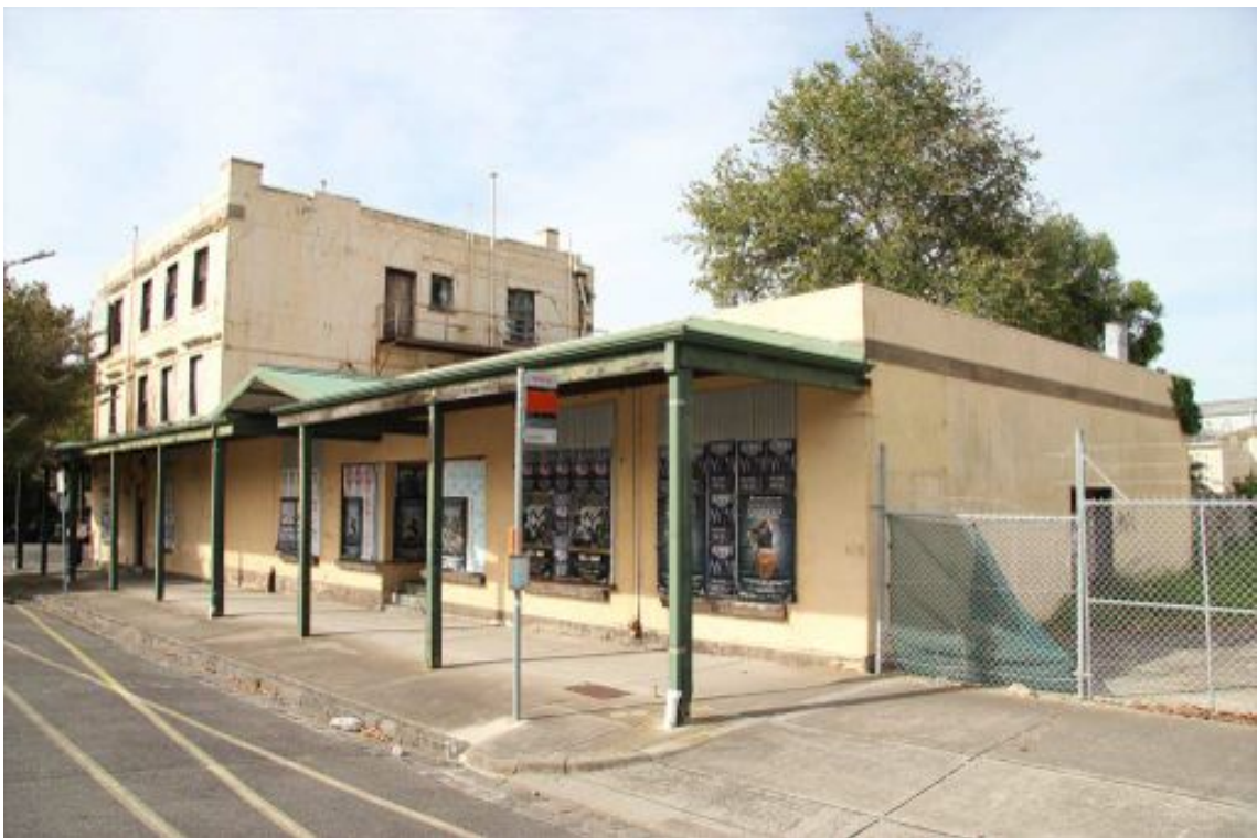
Figure 15 View of the hotel looking north, showing the later addition.
