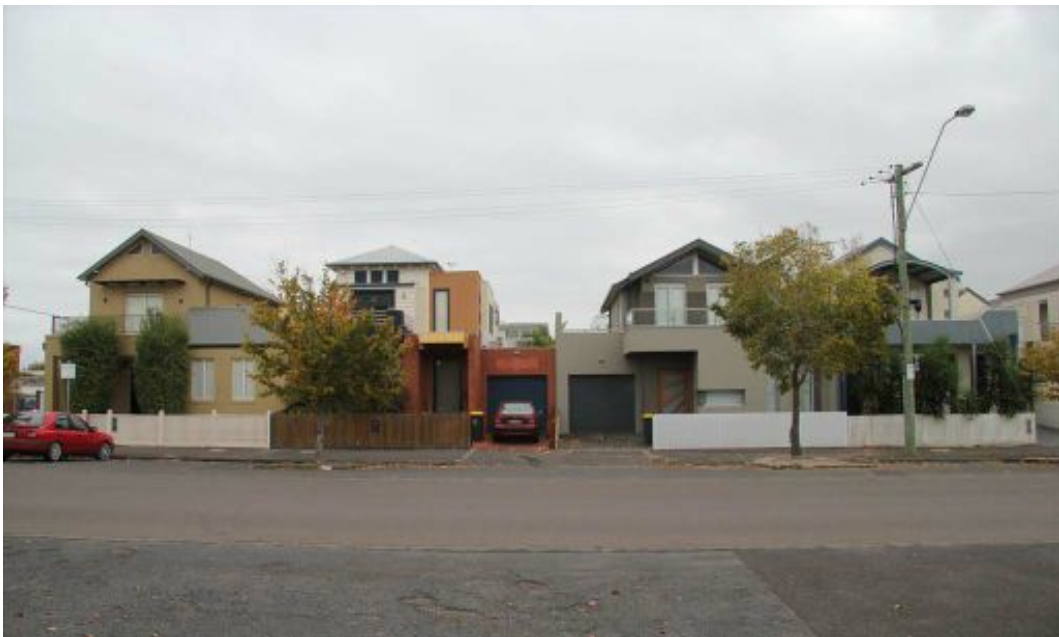
Figure 23 Residential development opposite the subject site in Ann Street.
