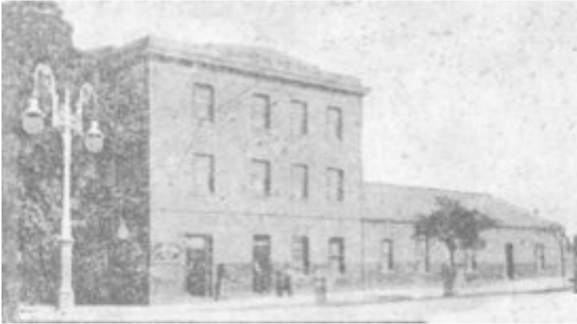
Figure 8 The Ann Street elevation of the Oriental Hotel, 1904. Source: Williamstown Illustrated .
