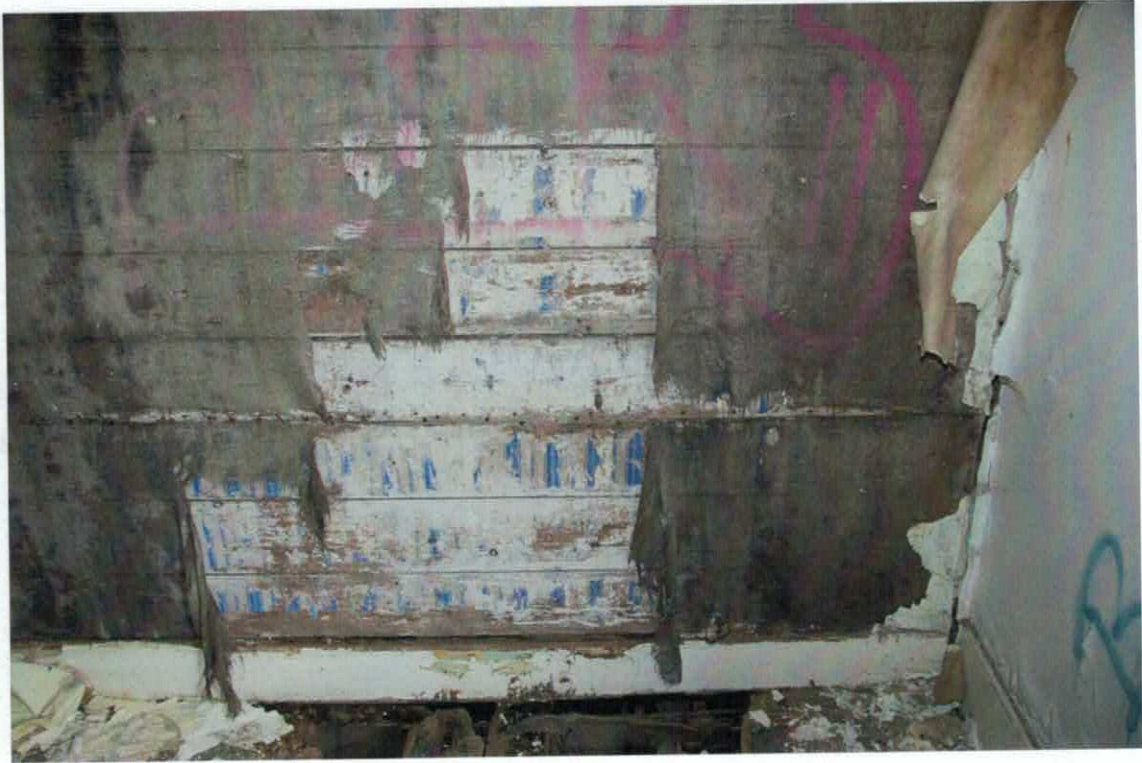
Figure 15 Detail of later timber framed partition wall on the second floor.
