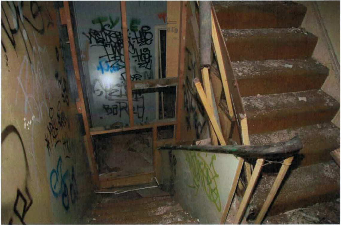
Figure 17 The stair between the first and second floors
