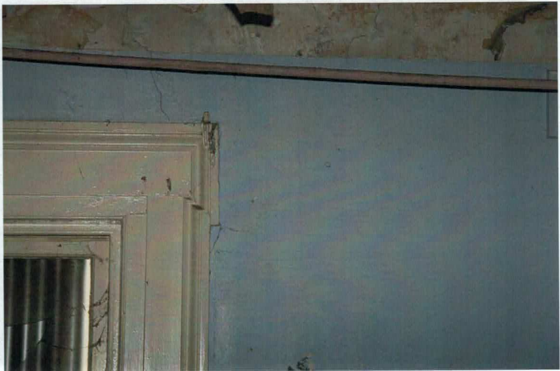
Figure 14 The architrave detail on the first floor
