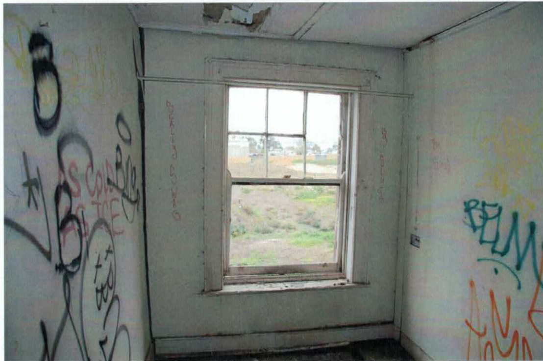
Figure 20 A single bedroom on the second floor showing the one surviving 6 pane window sash
