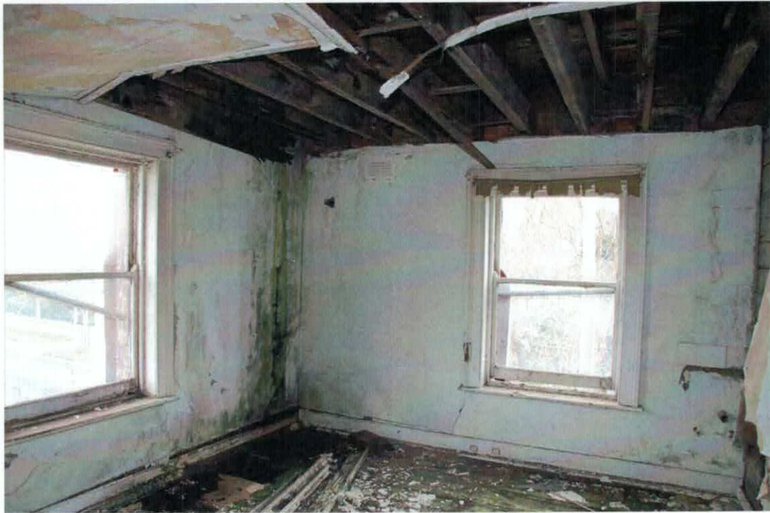
Figure 19 The second floor corner room
