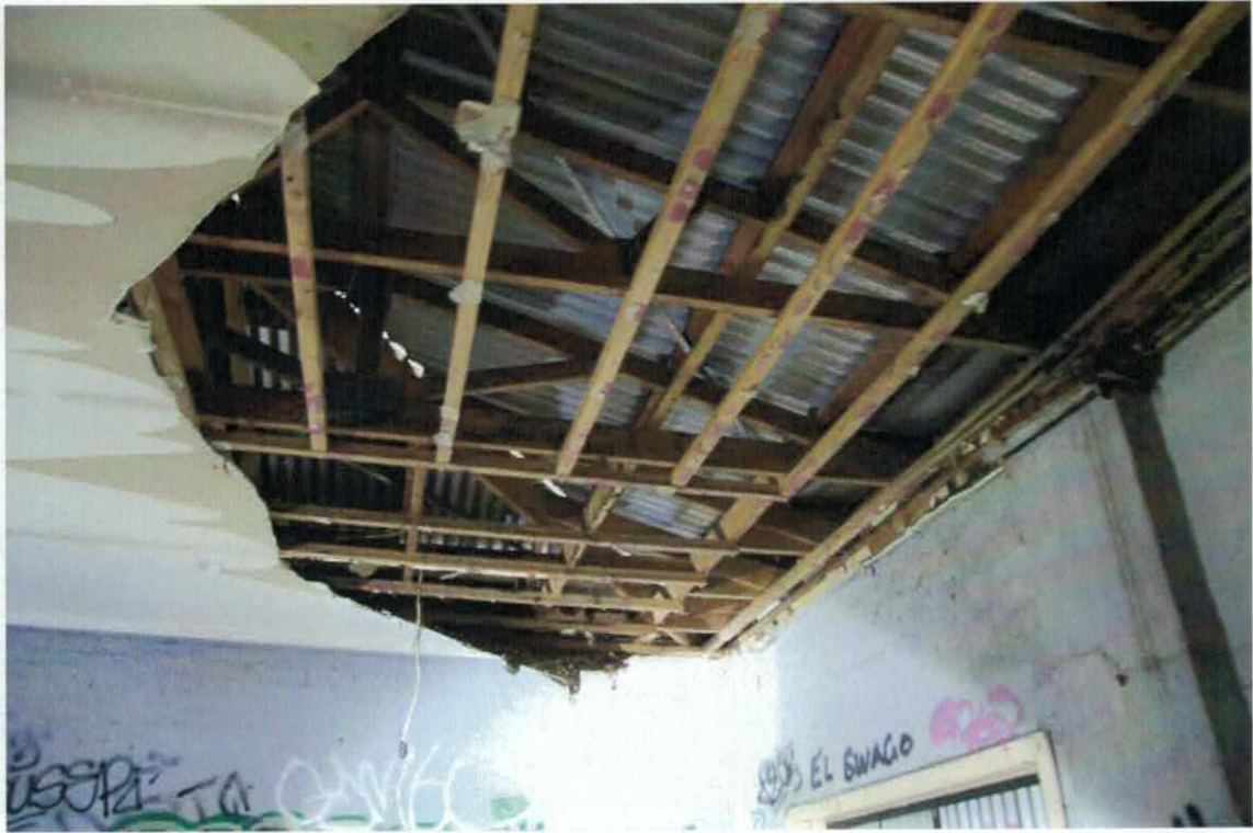
Figure 7 The roof framing to the Ann Street wing
