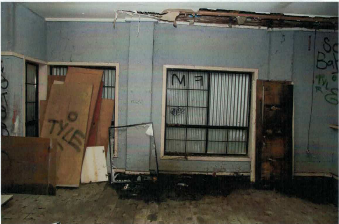
Figure 6 Detail of the Ann Street wall in the single storey wing
