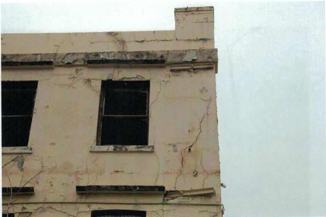
Figure 4 Detail of an upper level window
